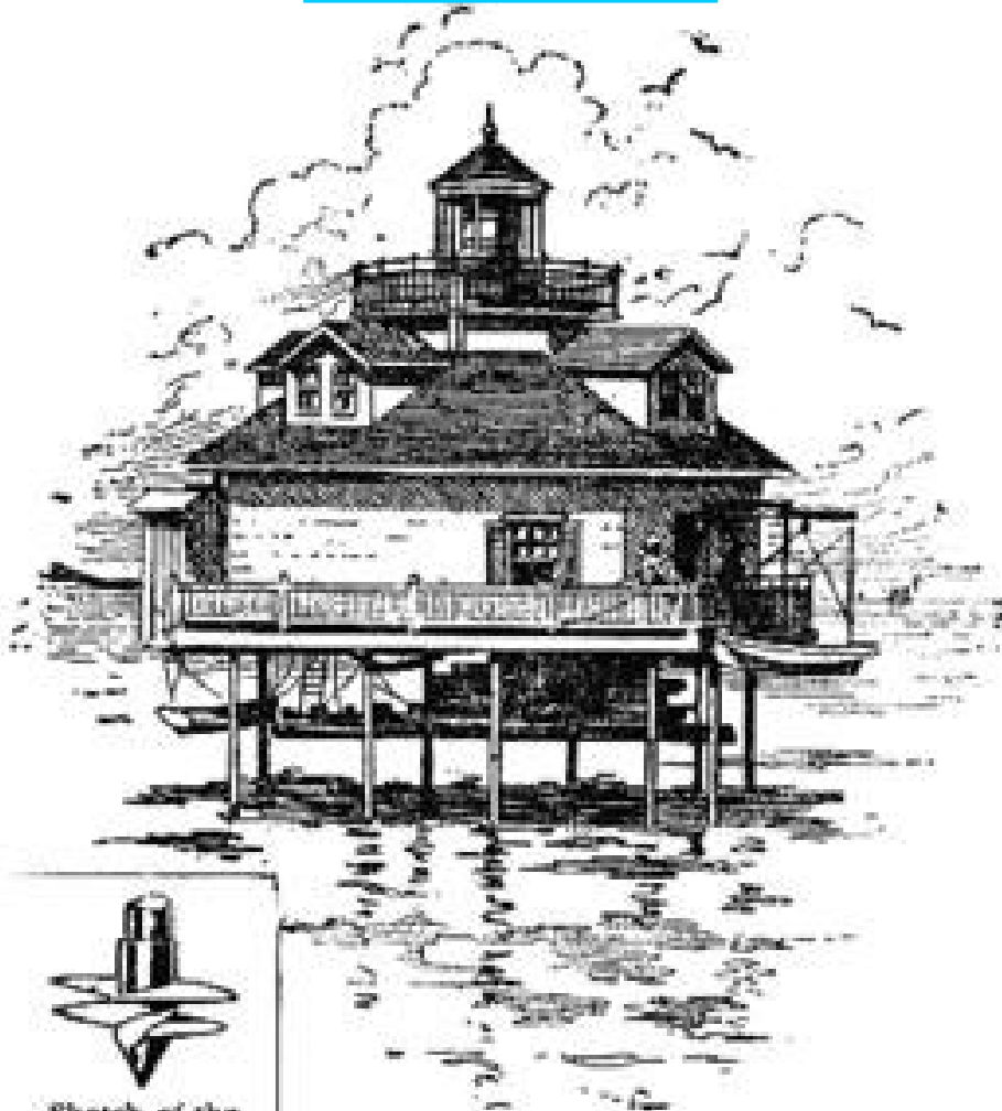
Sketch of the screw at the end of the pile
